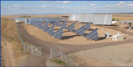
Prescott Airport, Single Axis, Tilted Tracker Single Axis and High Concentration Photovoltaic
