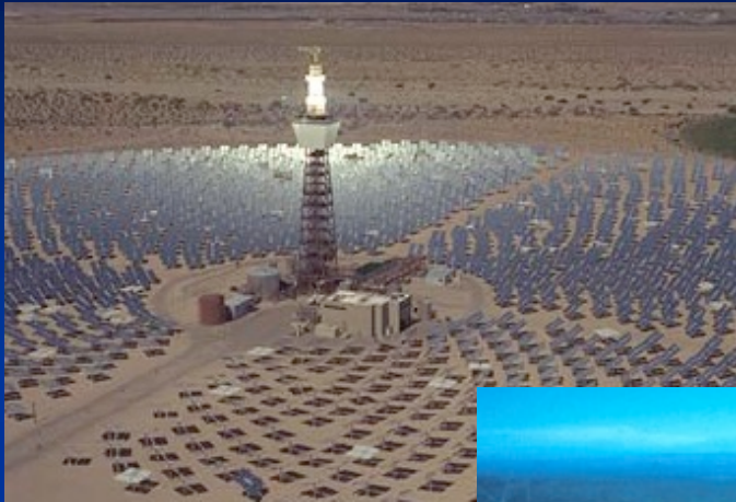
10 MW Solar II Experimental Power Plant, California
