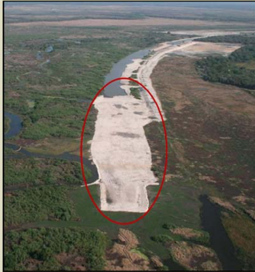
Backfilling of C-38 Canal March 2007
