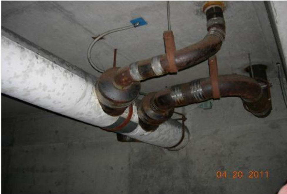
Figure 7 - Existing drainage system collecting rainwater from all levels and draining it to local sewer system.
