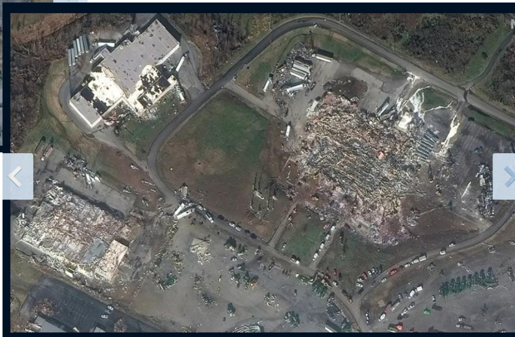
10_Overview of Mayfield consumer products candle factory and nearby buildings after tornado (Mayfield, Kentucky) 11dec2021
