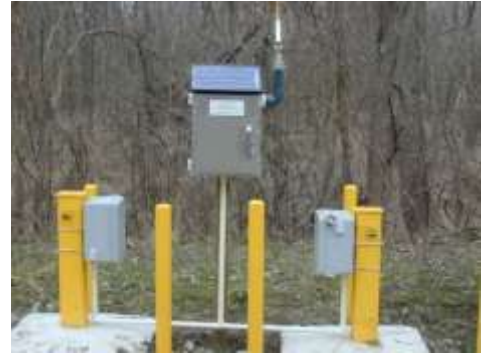
Ground water monitoring wells. Credit: U.S. Geological Survey (USGS)
