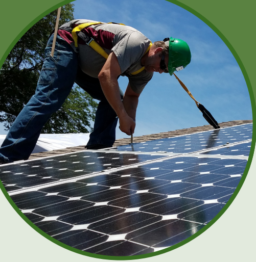
Faculty who attend the CREATE Energy Institute learn how to install solar photovoltaic panels.
