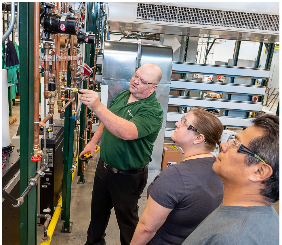
An HVAC instructor and students review hydraulic balancing and mixing for radiant floor heating.
