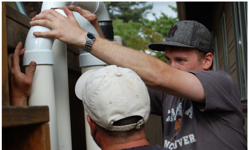
A WATER-I student attaches rainwater catchment system pipes with guidance from a local professional.
