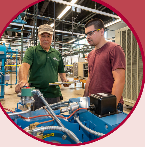
An instructor guides a student through the boiler inspection protocol in BEST's model curriculum.
