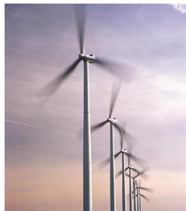
Public Service of Colorado Ponnequin Wind Farm. Credit: Warren Gretz/NREL
