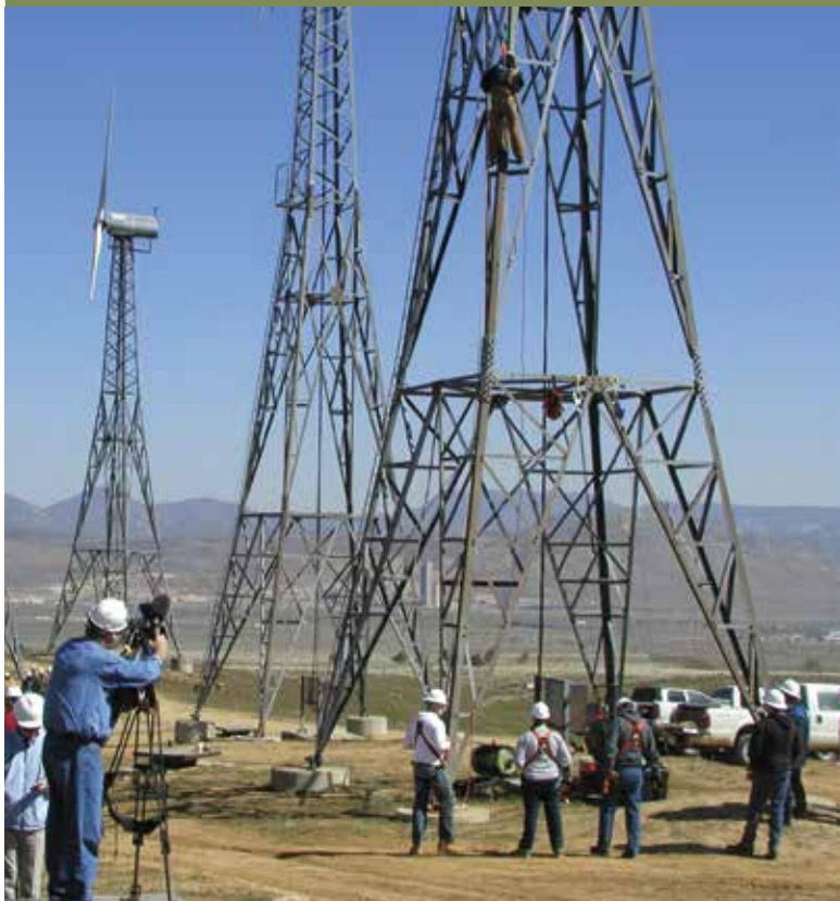
Wind turbine technicians prepare to climb the turbine tower.
